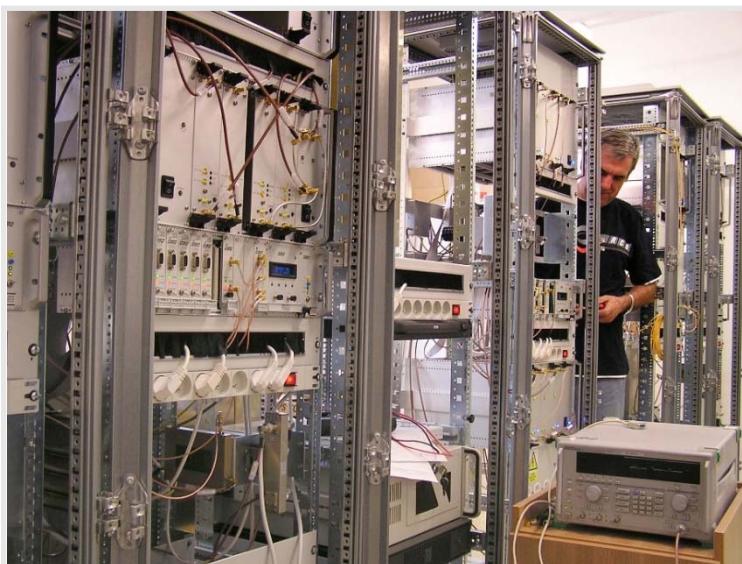
Road Tunnel Technology Assembling
