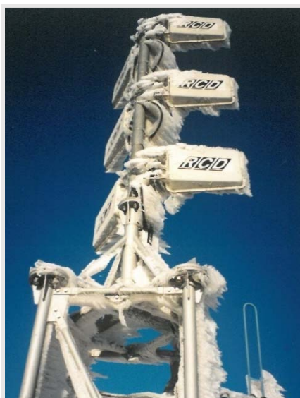
Antennas of TETRAPOL Radio System
